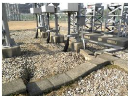
Okuma line 3L, Ground wire (disconnected)
