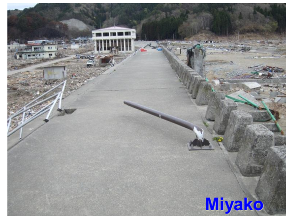
Destruction by wave pressure
