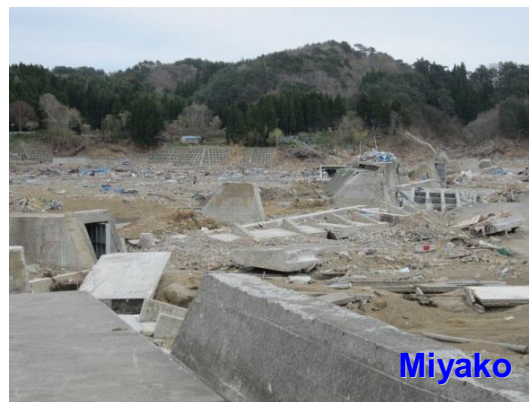
The 10m-high seawall was destroyed in Taro district, Miyako city, Iwate Pref.
