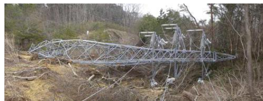
Collapsed tower
