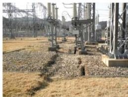
Okuma line 3L, Ground wire (disconnected)
