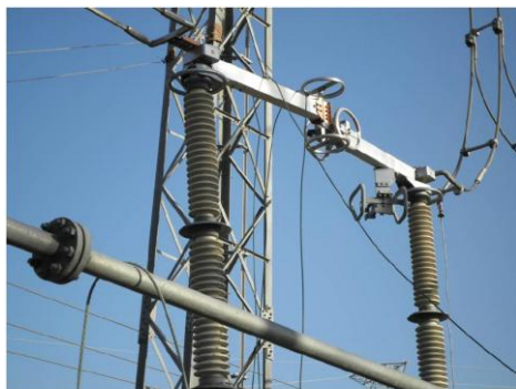
Okuma line 3L, Ground wire (disconnected)
